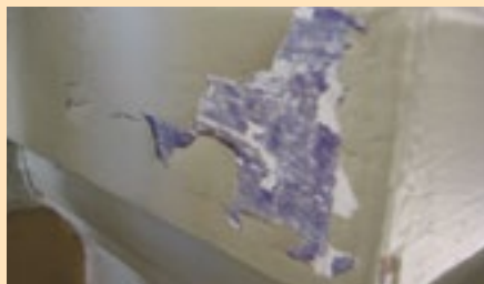
Small portions of damage to the current paintwork suggest that some fixtures in the room were once painted bright blue
