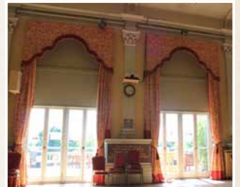
By 2019 the whole room, including the windows, was in desperate need of repair.
